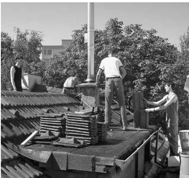
Josh, Mike, Rodion, Jelico. Dacharbeiten 2006
